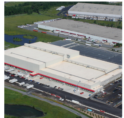
Chester, N.Y. Facility
