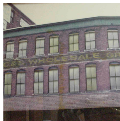
Early C&S Warehouse
